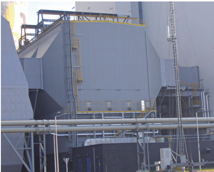
FIGURE 1: A recently commissioned Alstom electrostatic precipitator placed after an 850 MW lignite-fired boiler in Poland.
